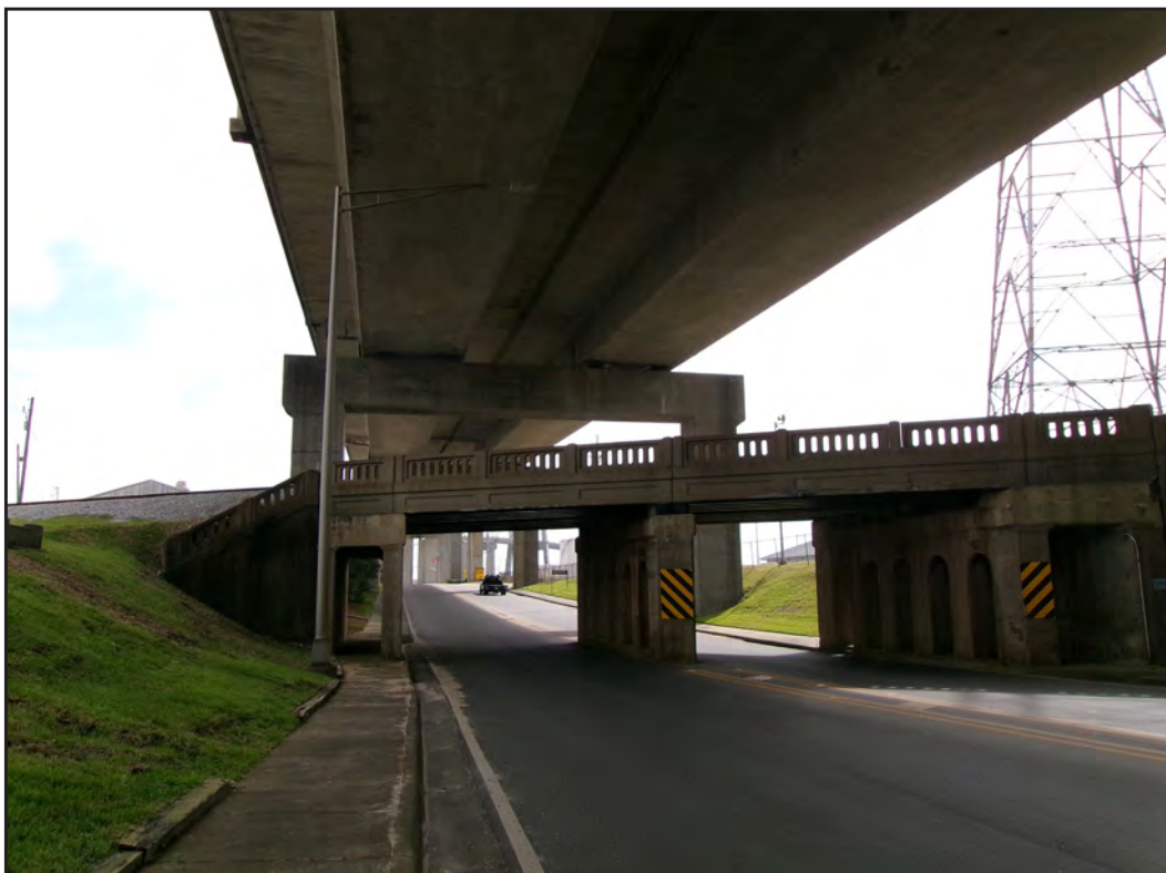
Figure 6. View of railroad bridge passing under Africatown Boulevard, facing east.
