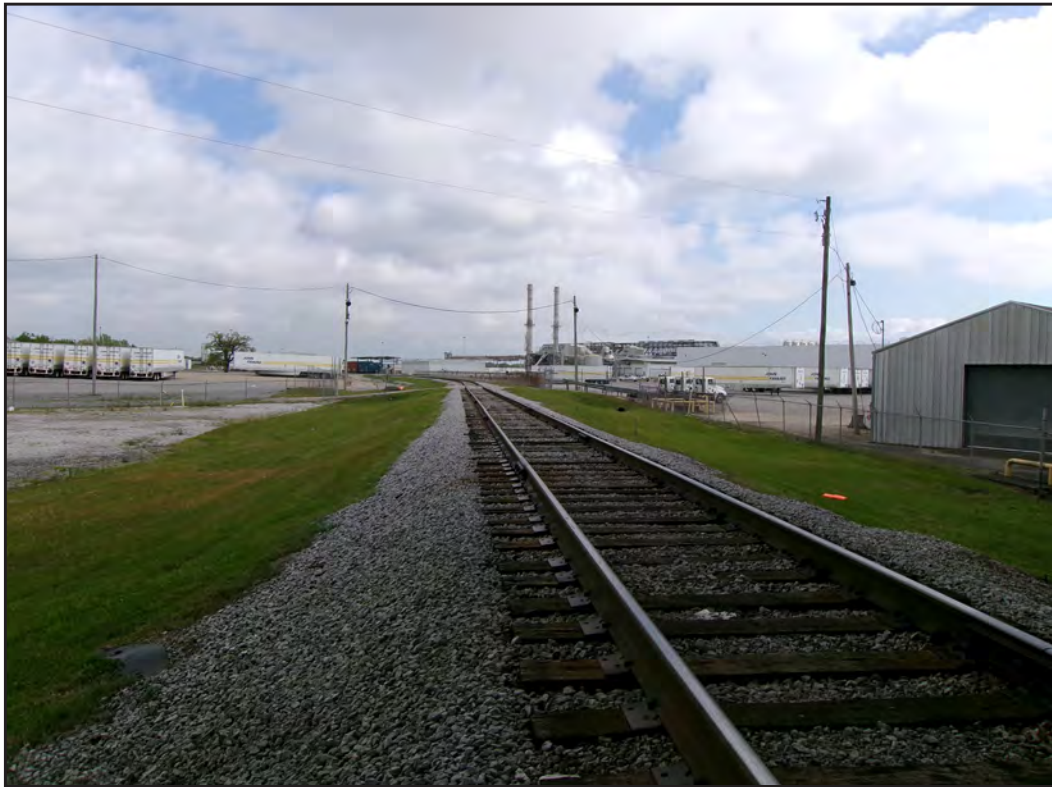
Figure 5. View of tracks adjacent to Kimberly-Clark facility in central portion of LOD, facing north-northeast.
