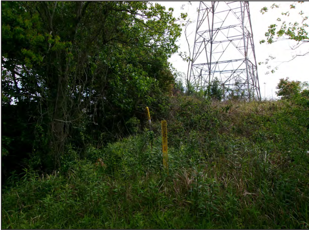
Figure 11. View of buried utility postings in the central LOD, facing east.
