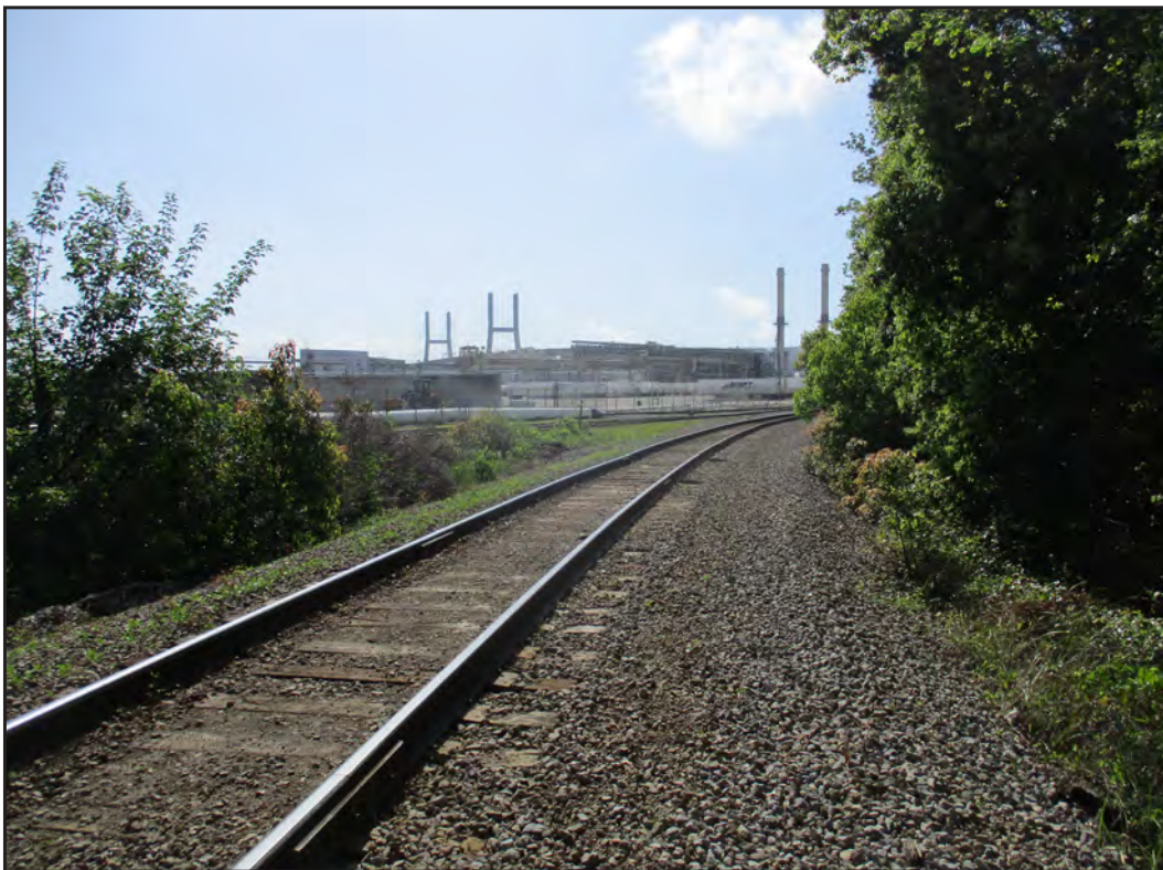
Figure 12. View of central LOD from Berg Spiral Pipe facility, facing southeast.
